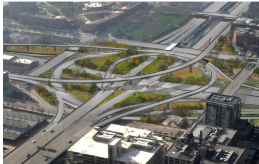
Artist’s rendition of renovated Jane Byrne Interchange, facing west. Map source: Illinois Transportation and Highway Engineering Conference.
